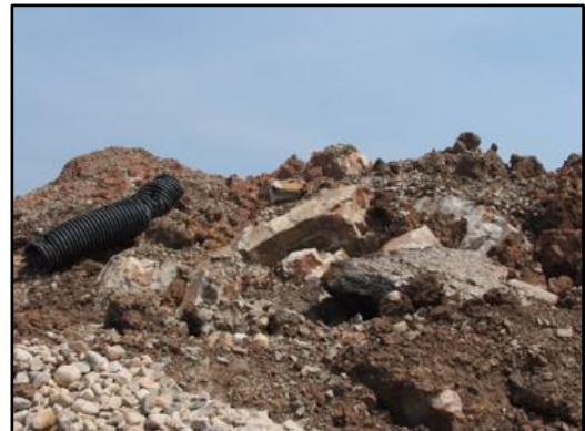
Old storm sewer basin and edge drains await collection.
